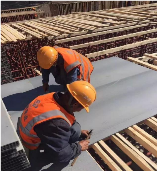
Roof Form Erecting
