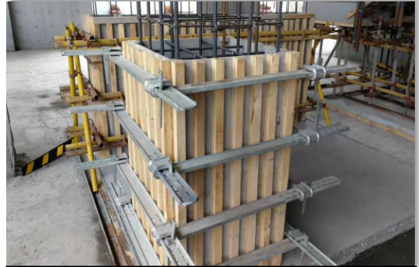
Column Form Erecting
