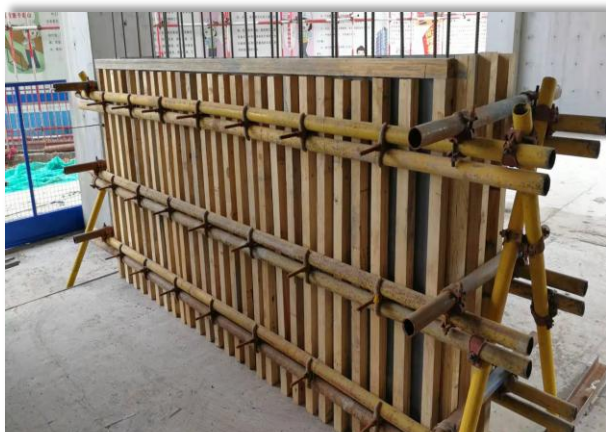
Wall Form Erecting
